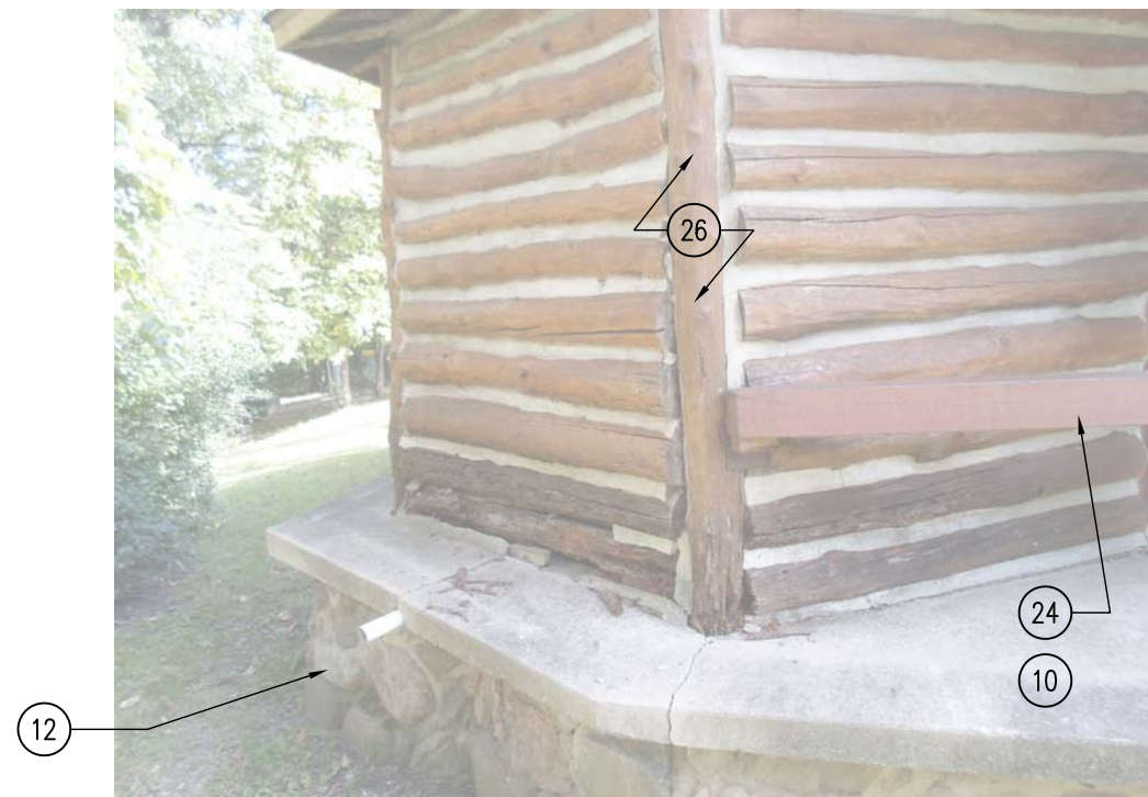
01 PUMP HOUSE PICTURE - SLAB, WALL, AND LOGS SCALE: NTS
